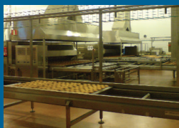
TWO COMPLETE LINES WITH A CAPACITY OF 30,000 UNITS PER HOUR.
